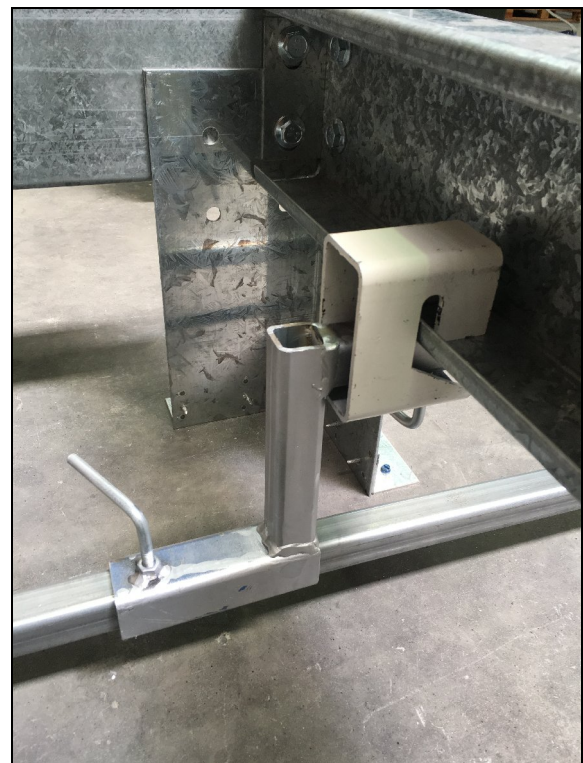
Figure 2: Offset bracket (Z design) with C-purlin clamp
